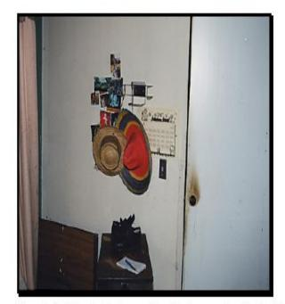
Figure 7 - Interior of patient room, where the door was closed during the fire (NFPA)
